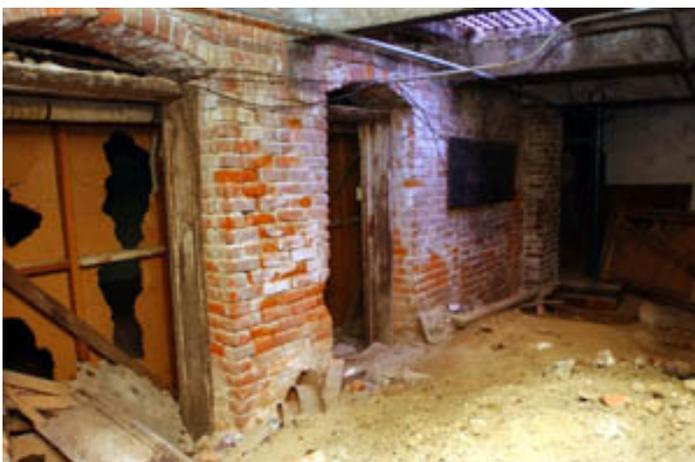
**Original storefront and ground level; the girders above support the elevated present-day sidewalk**
