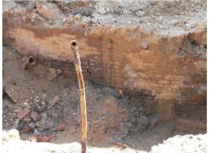
Pictures 3-4 are of construction/repairs around a pipe at Gibbon and South Royal Streets (near the Safeway, for those familiar with the area). Note that the main pipe is made of bricks.
